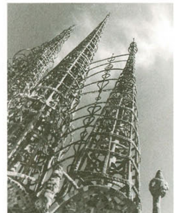
SIMON RODIA Watts Towers, 1955
